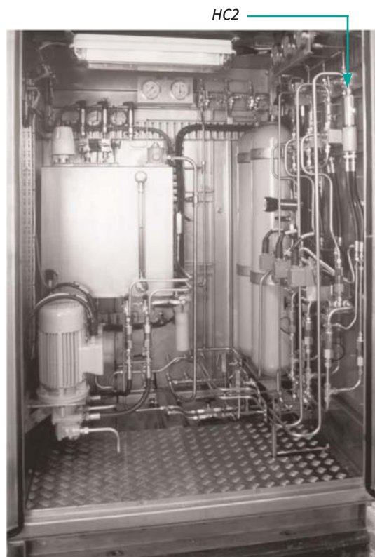
Well Control Panel
